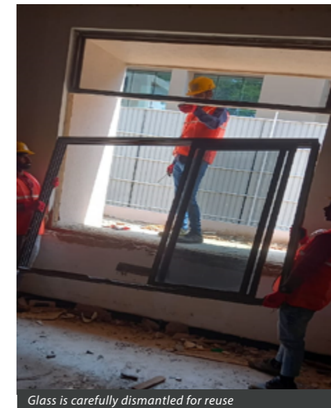
Glass is carefully dismantled for reuse
