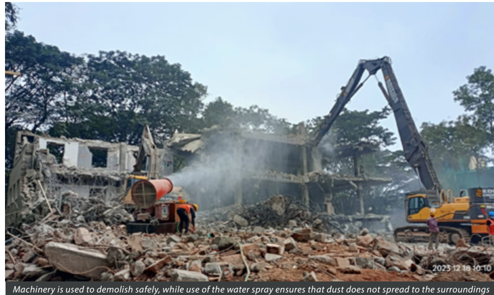
Machinery is used to demolish safely, while use of the water spray ensures that dust does not spread to the surroundings
