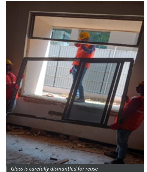
Glass is carefully dismantled for reuse
