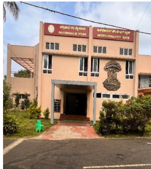
Figure 110: Infosys Foundation block at Shakthidhama
