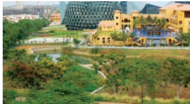
Rain water harvesting at Infosys
