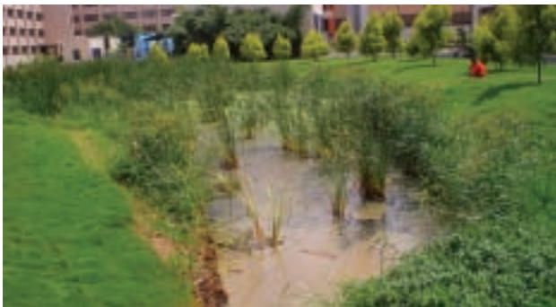
Rain water harvesting at Infosys
